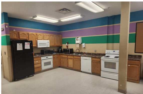
Above: The Omaha Cares program kitchen before the remodel.
