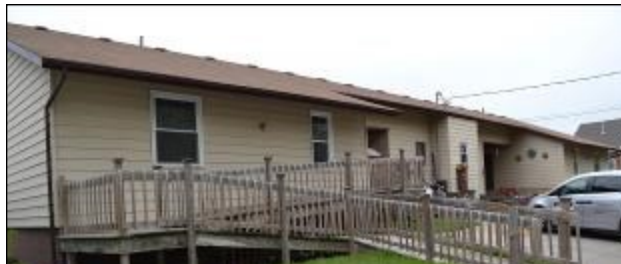
4th Street Duplex has undergone major renovations
